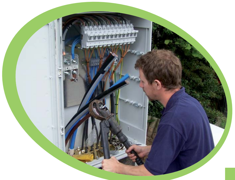
Distribution unit installation
